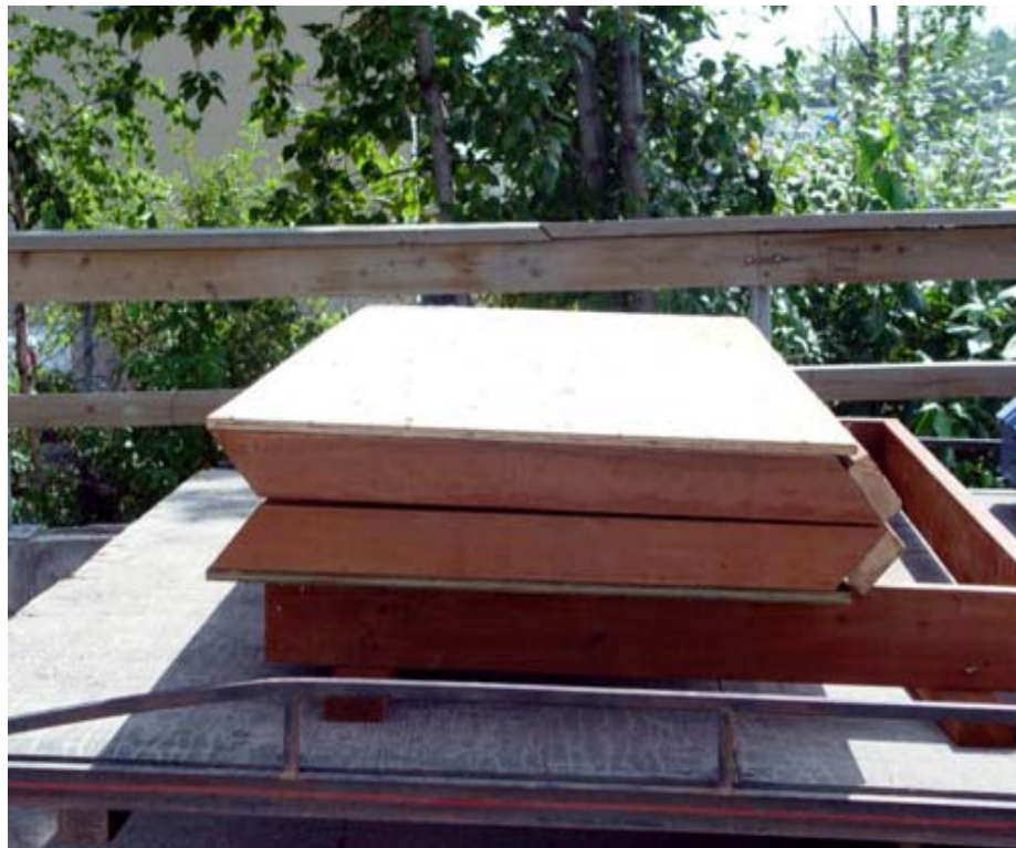
Photo 3: Plywood roof panels before shipment to the village.
