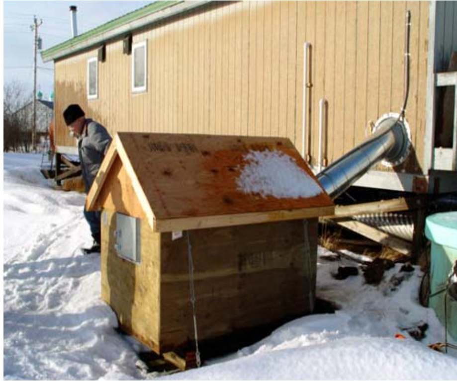
Photo 2: Premanufactured plywood roof panels installed.
